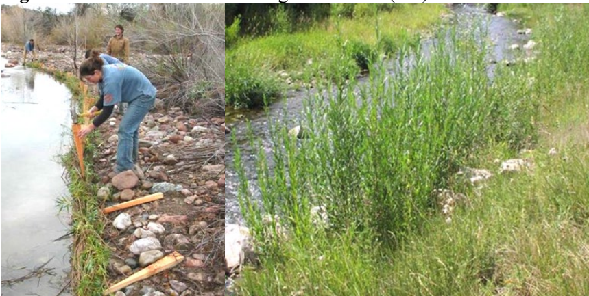
Figure 16-12: Live Fascine during Installation (left) and after Establishment
