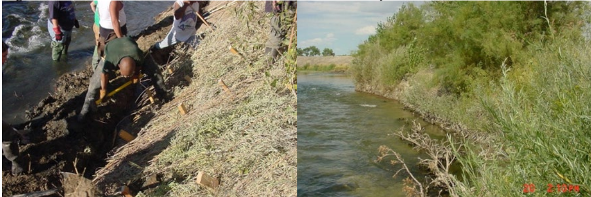
Figure 16-2: Brush Mattress. Under construction and after 2 years.
