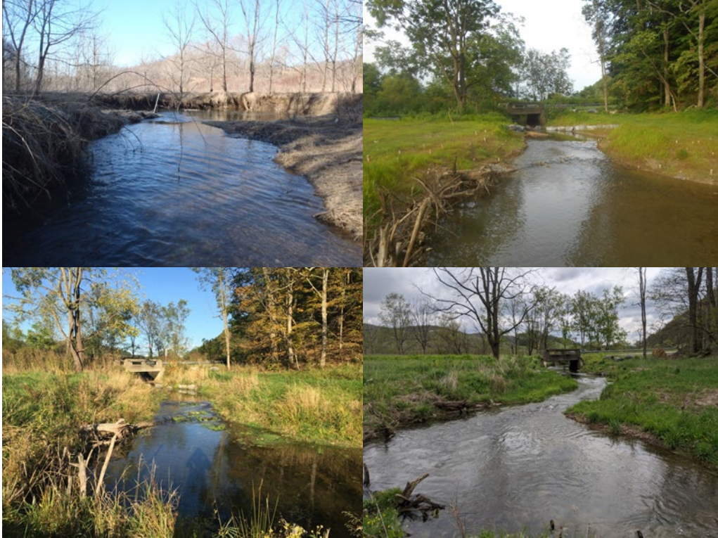
Figure 16-18: Rootwad Revetment with Bank Grading before Installation (top left), immediately after Installation (top right), after two years (bottom left), and after five year (bottom right)
