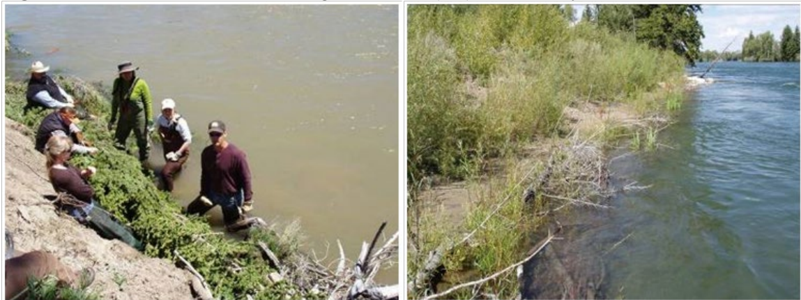
Figure 16-14: Brush Revetment during Installation (left) and after 2 years
