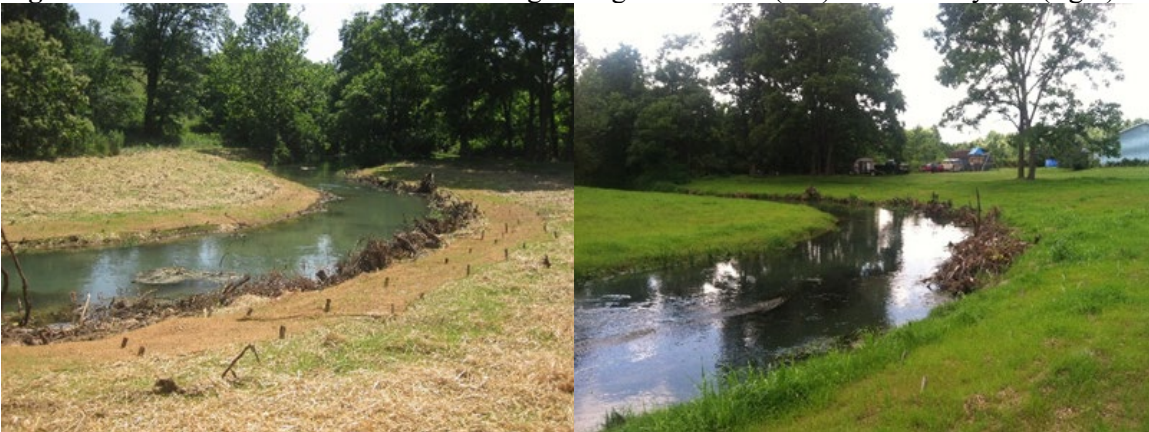
Figure 16-17: Toe Wood with Bank Grading during Installation (left) and after 2 years (right).
