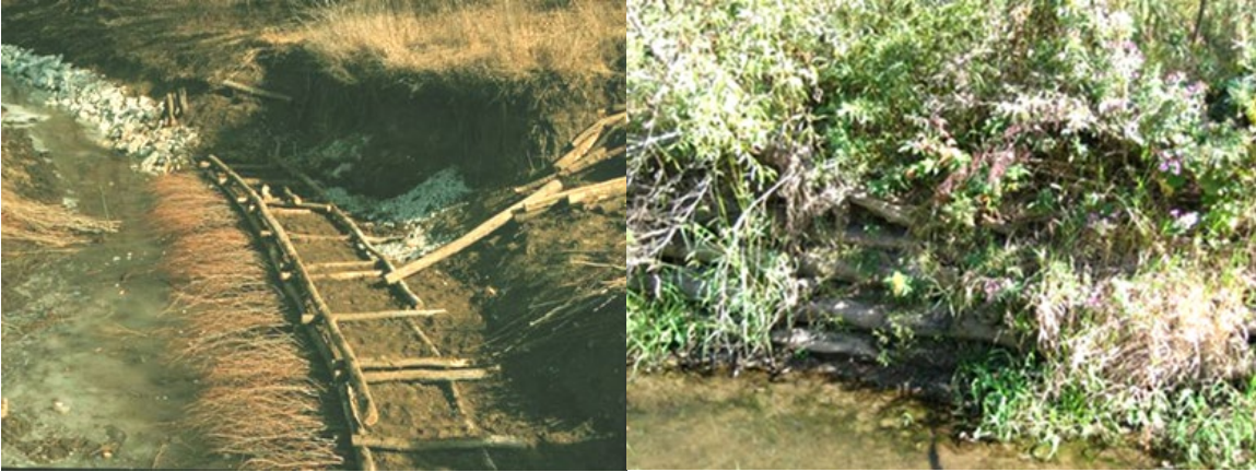
Figure 16-13: Live Cribwall during Installation (left) and after 10 years
