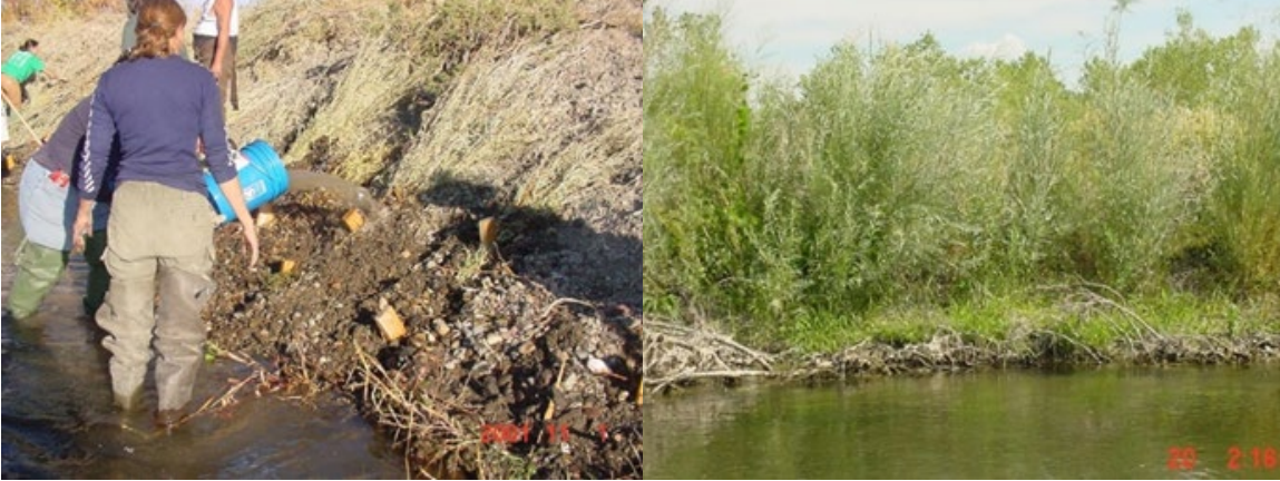
Figure 16-16: Vertical Bundles with Brush Revetment during Installation (left) and after 2 years
