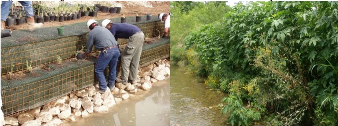
Figure 16-1: Vegetated wire face MSE wall. Under construction and after 2 years.
