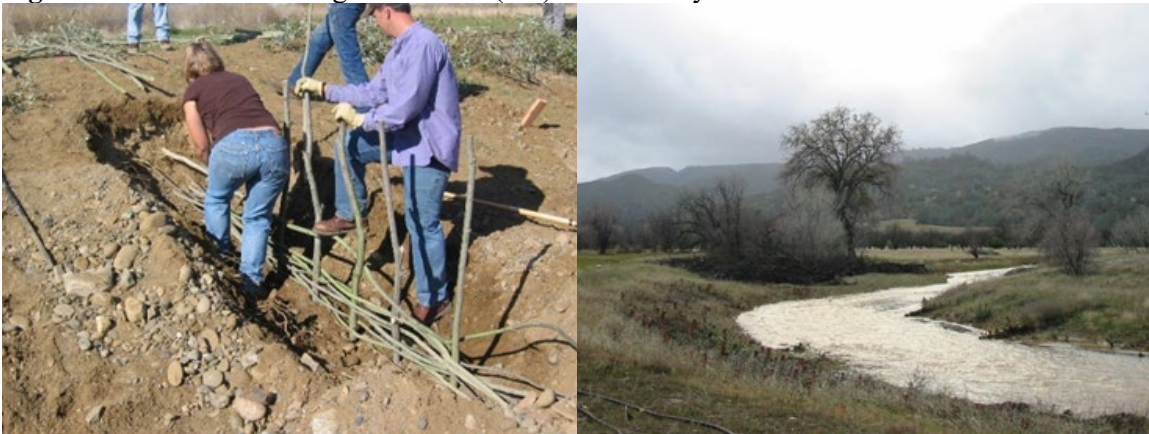
Figure 16-15: Wattle during Installation (left) and after 2 years
