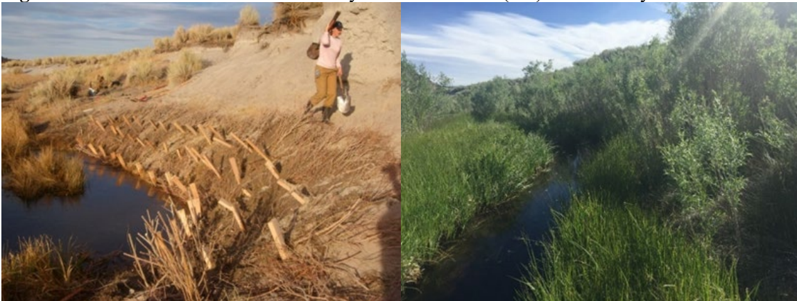
Figure 16-11: Brush Mattress immediately after installation (left) and after 9 years.
